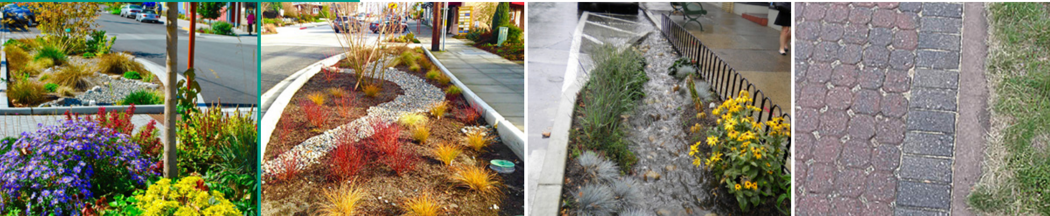
Left to Right: Two colorful rain gardens to help manage stormwater in Langley, Washington. PHOTOS BY LANGLEY MAIN STREET ASSOCIATION, COURTESY OF WASHINGTON MAIN STREET AND THE WASHINGTON TRUST FOR HISTORIC PRESERVATION. Curb cut-out inlet to Allen Street Rain Gardens in State College Borough, Pennsylvania. PHOTO BY STATE COLLEGE BOROUGH. Permeable pavers. PHOTO BY U.S. EPA
