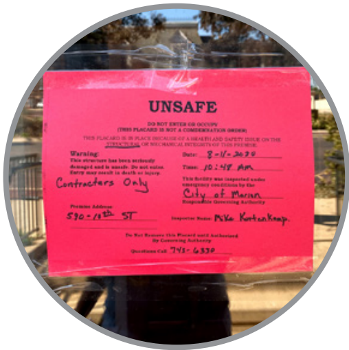
A structure in Marion, Iowa, is deemed unsafe to enter after the derecho in 2020. PHOTO BY UPTOWN MARION
